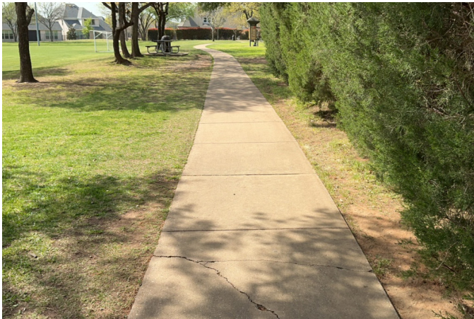
Harmony Park: Perimeter Concrete Sidewalk
