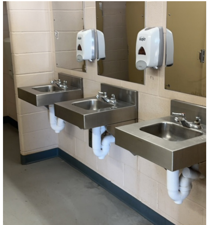
Independence Park East: Restrooms
