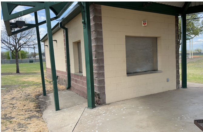
Independence Park West: Concession Building
