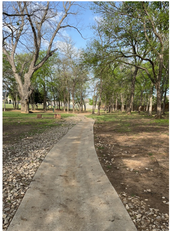
Freedom Dog Park: Drainage Concrete Channel
