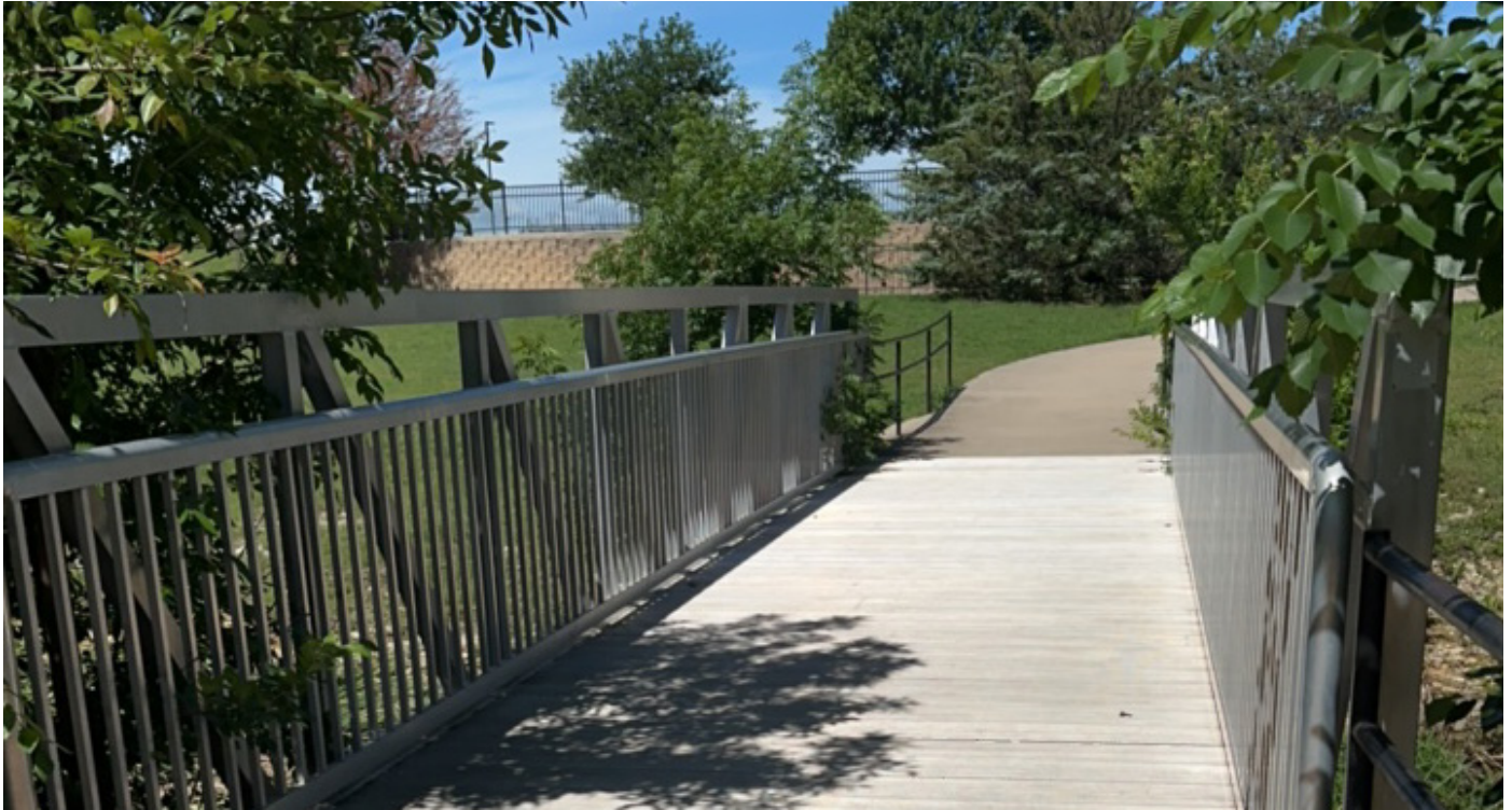
Linear Park Trail: Utility Bridge
