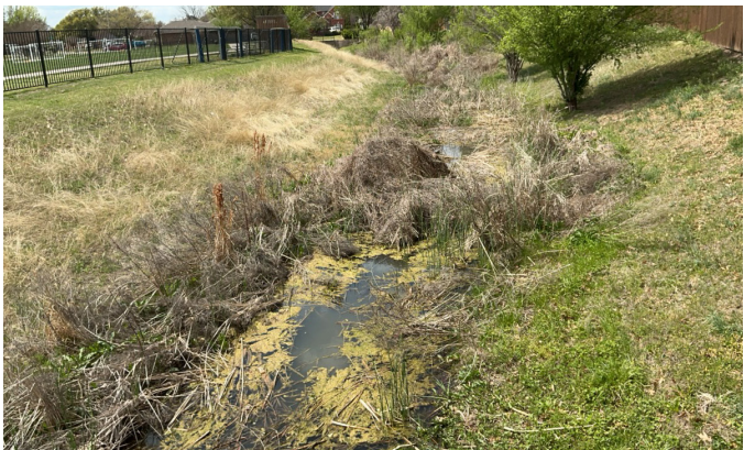
Lakeview Park Trail: Under Utility Bridge
