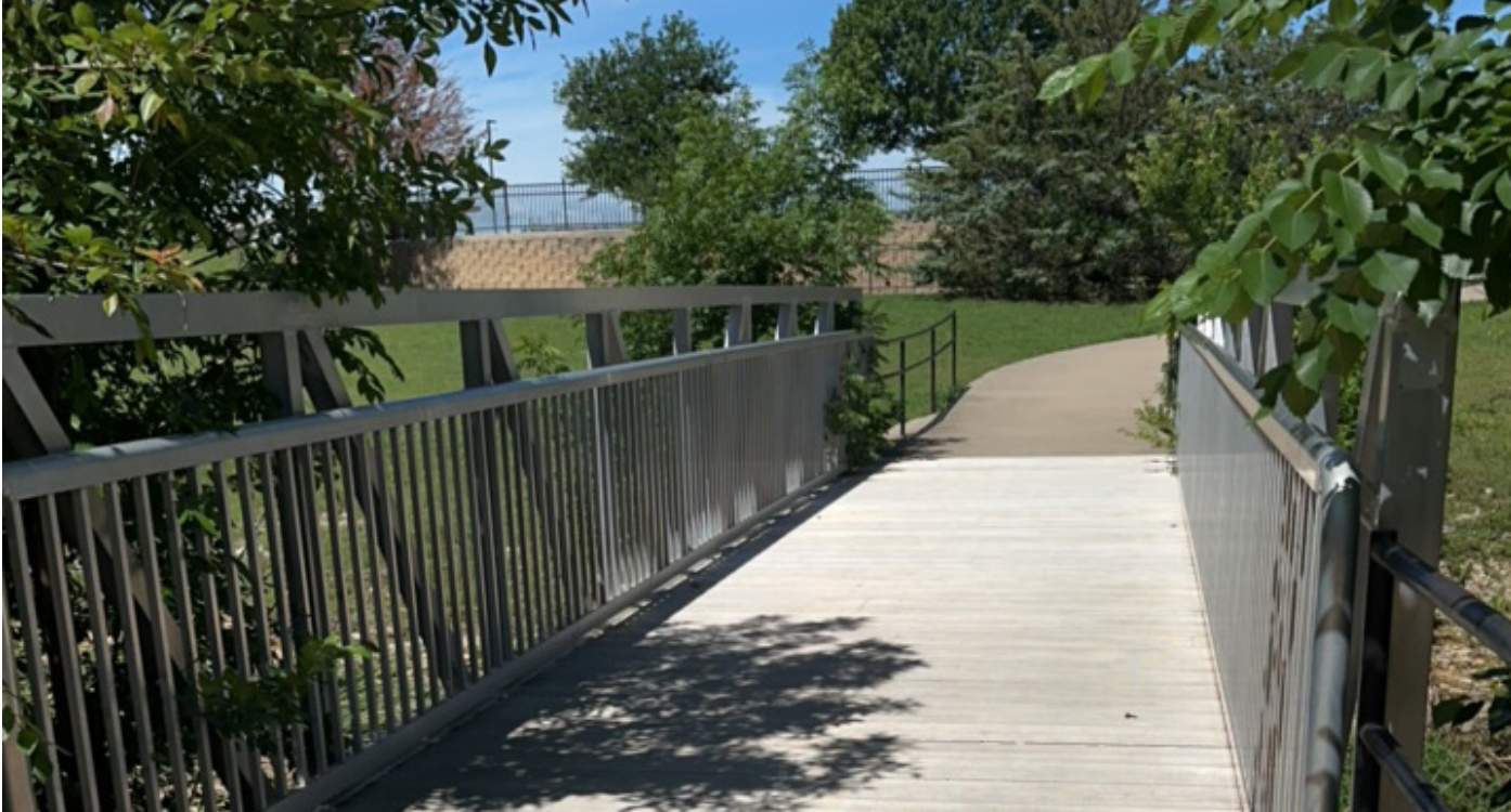
Linear Park Trail: Utility Bridge
