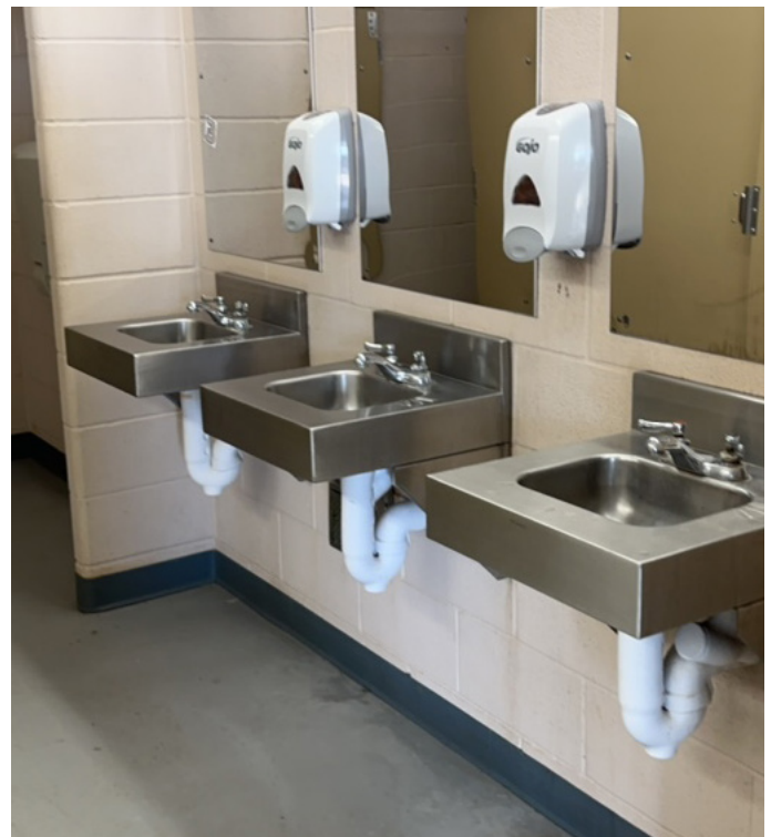
Independence Park East: Restrooms
