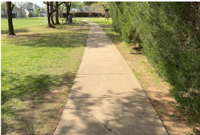
Harmony Park: Perimeter Concrete Sidewalk
