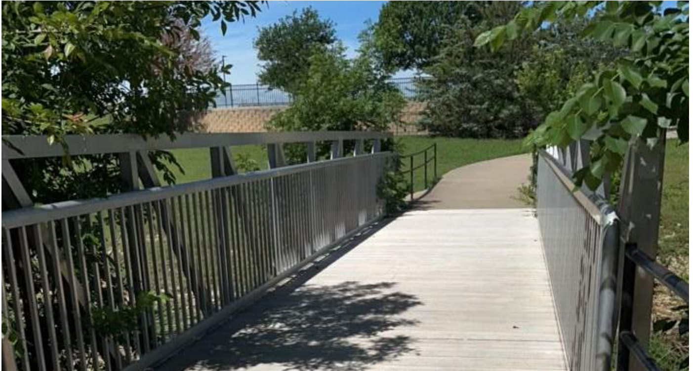
Linear Park Trial: Utility Bridge
