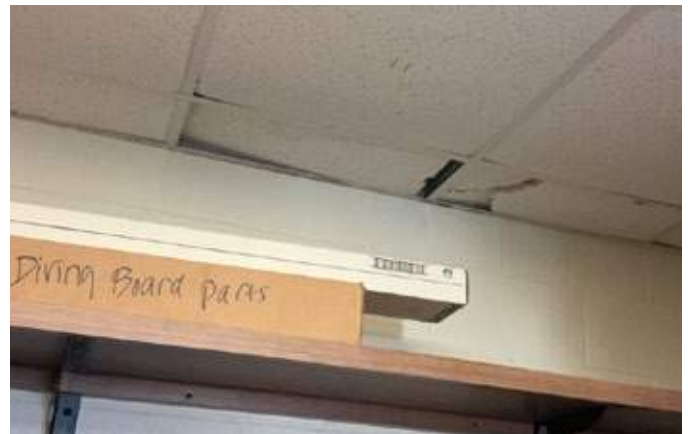
Independence Park East: Community Pool Storage Room
