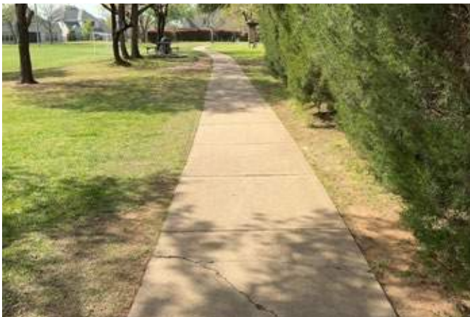
Harmony Park: Perimeter Concrete Sidewalk
