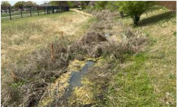
Lakeview Park Trail: Under Utility Bridge
