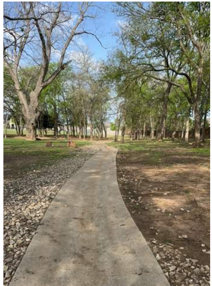
Freedom Dog Park: Drainage Concrete Channel
