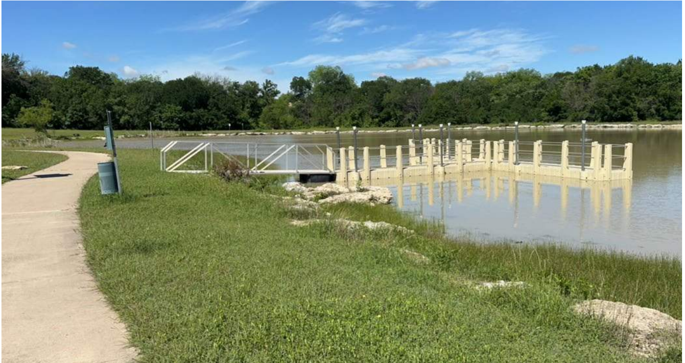
Linear Park: Pier Near Chatswood Drive
