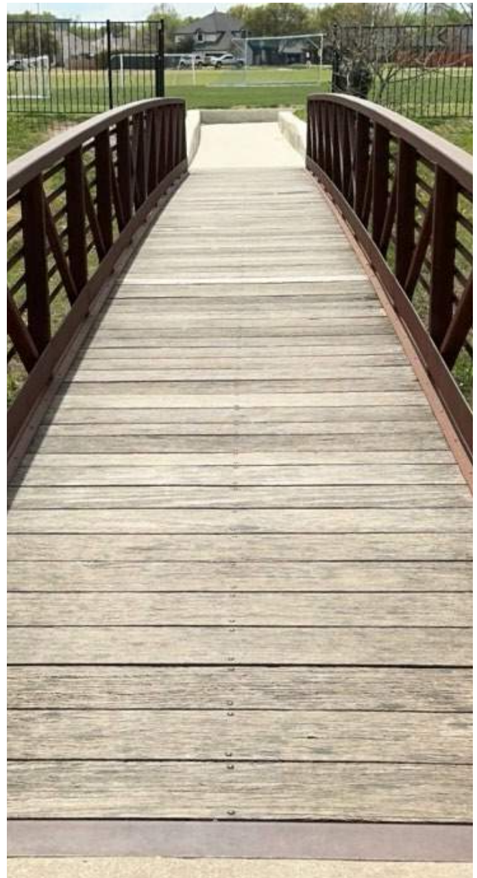
Lakeview Park Trail: Utility Bridge
