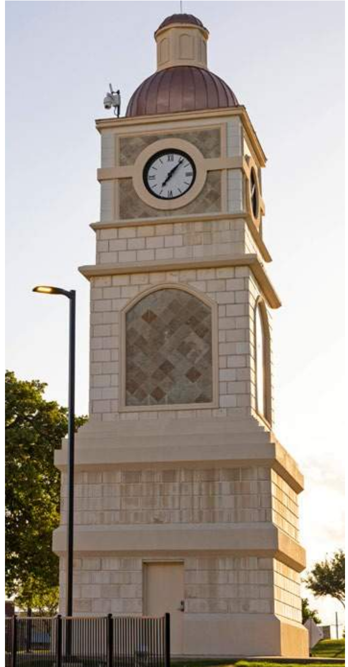
ToTC Clock Tower
