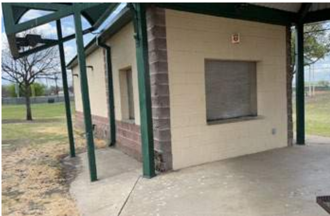
Independence Park West: Concession Building
