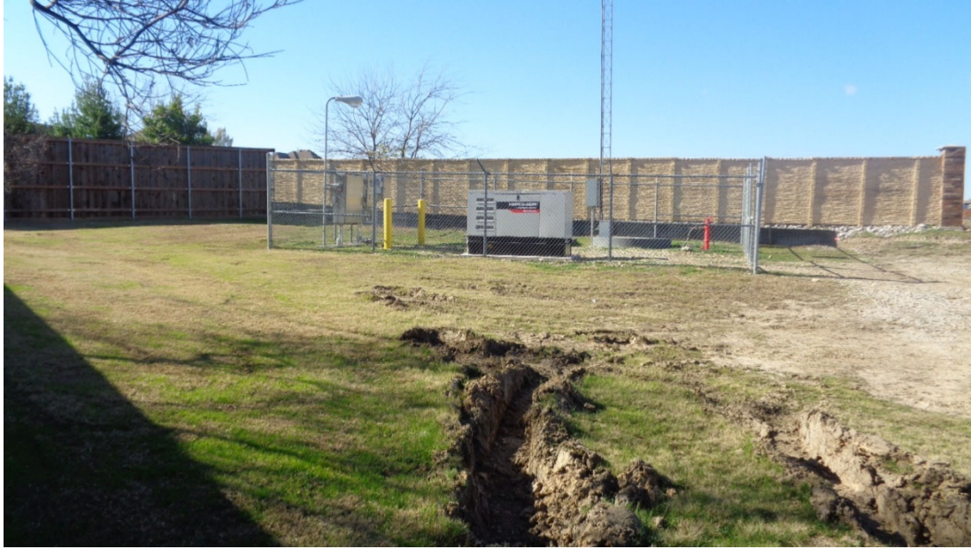
VIEW FROM NORTHERN PORTION OF THE SUBJECT LOOKING WEST AT SUBJECT PROPERTY (SEWER LIFT STATION NOT PART OF SUBJECT)
