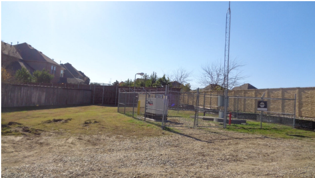
VIEW FROM NORTHERN PORTION OF THE SUBJECT LOOKING SOUTHWEST AT SUBJECT PROPERTY (SEWER LIFT STATION NOT PART OF SUBJECT)
