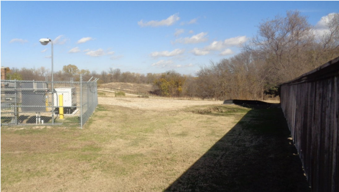
VIEW FROM SOUTHERN PORTION OF THE SUBJECT LOOKING NORTH AT SUBJECT PROPERTY
