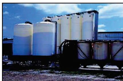
Large cone bottom tanks ranging in sizes from 2,500 to 13,000 gallons, are used to store and deliver up to 10,000 cubic ft. of bulk resins at a processing plant.
