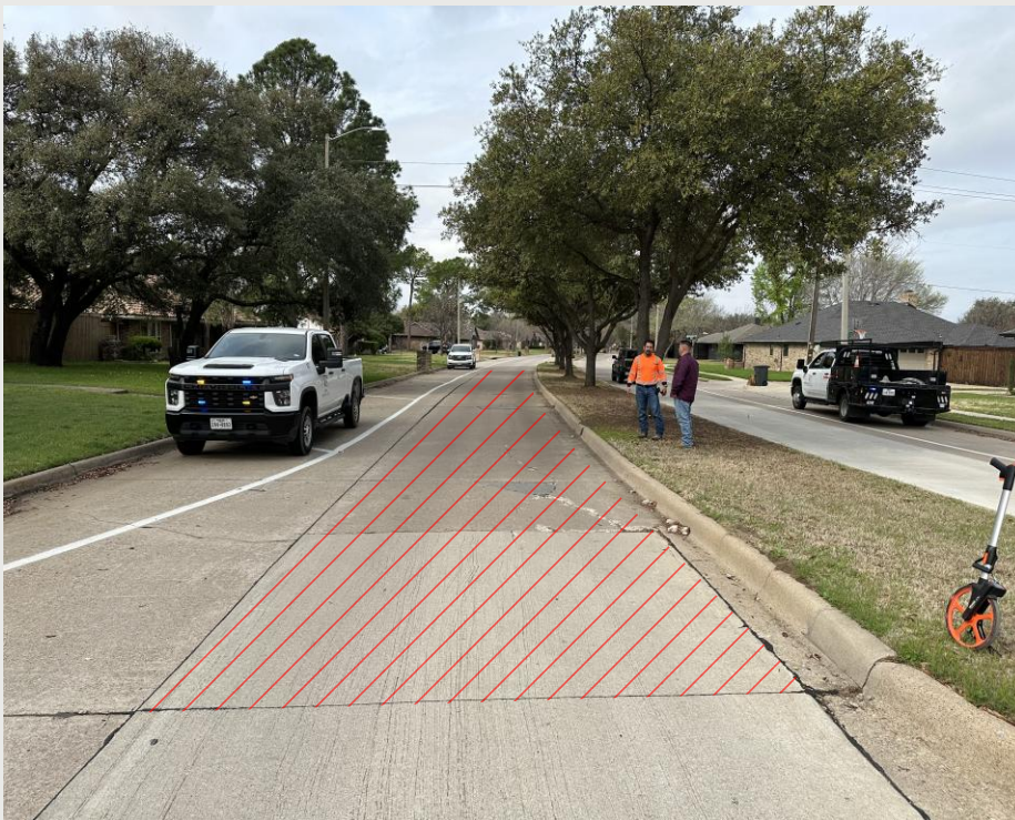
Area #1 - 8" Concrete: 212 X 12
