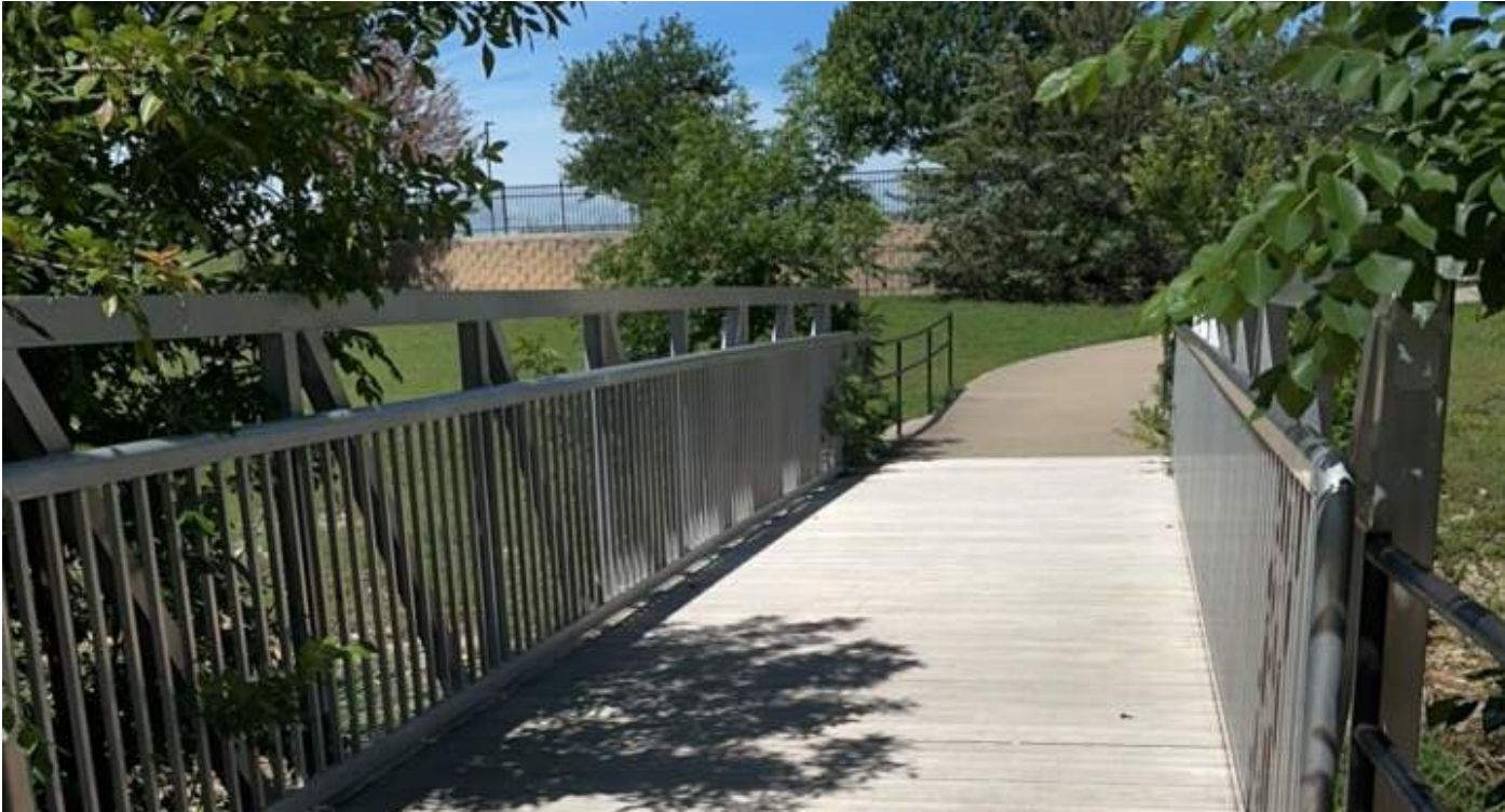
Linear Park Trail: Utility Bridge
