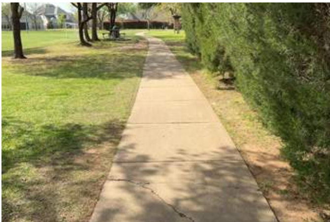
Harmony Park: Perimeter Concrete Sidewalk
