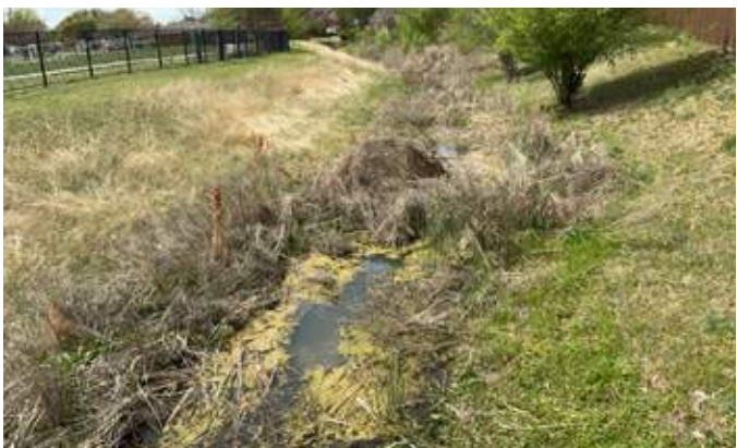
Lakeview Park Trail: Under Utility Bridge
