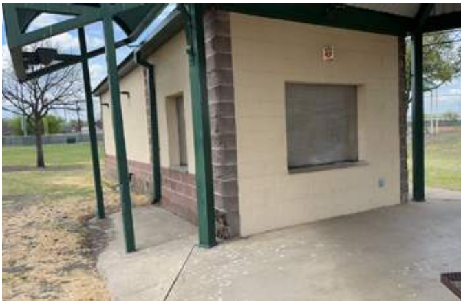
Independence Park West: Concession Building
