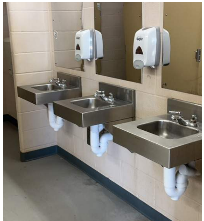
Independence Park East: Restrooms
