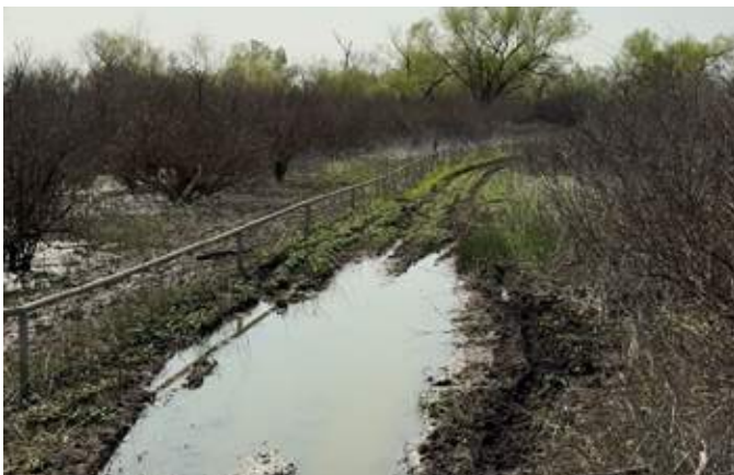
Trophy Club Park Trail: Flooding & Erosion
