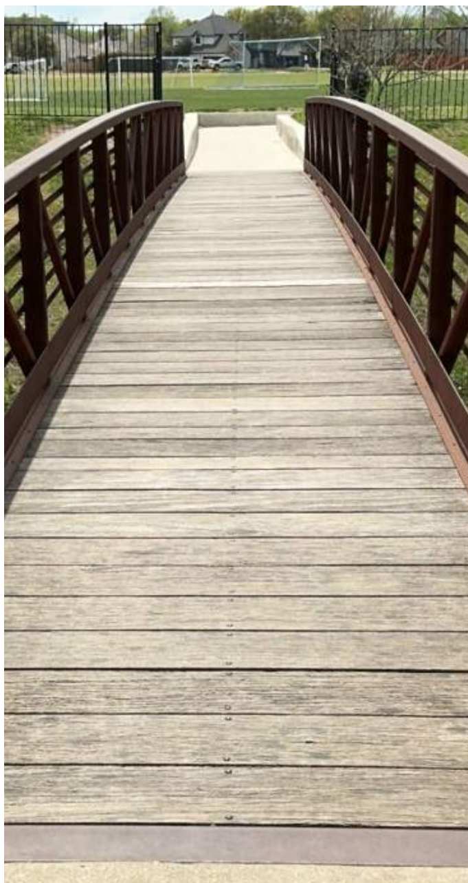
Lakeview Park Trail: Utility Bridge
