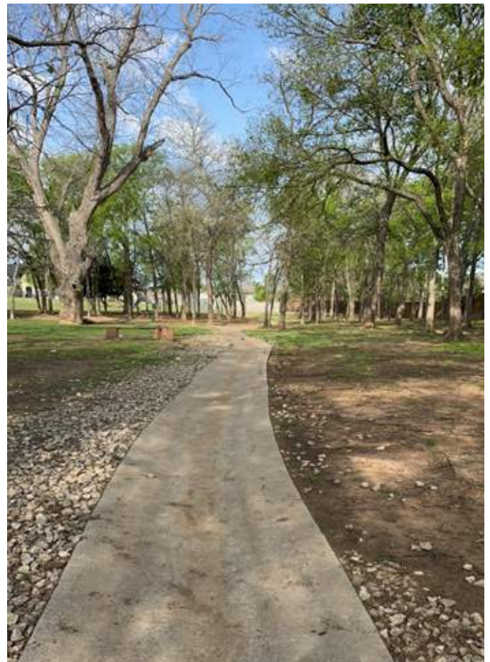
Freedom Dog Park: Drainage Concrete Channel
